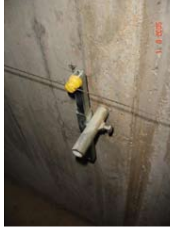
Figure 23: Stakes to support the stringlines fixed to the walls
