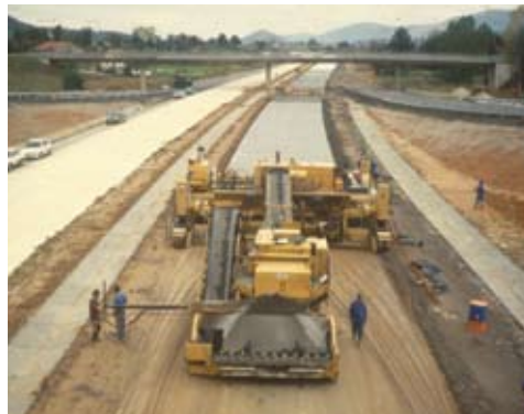
Figure 25: Mechanical steel placement in a continuously reinforced concrete pavement
