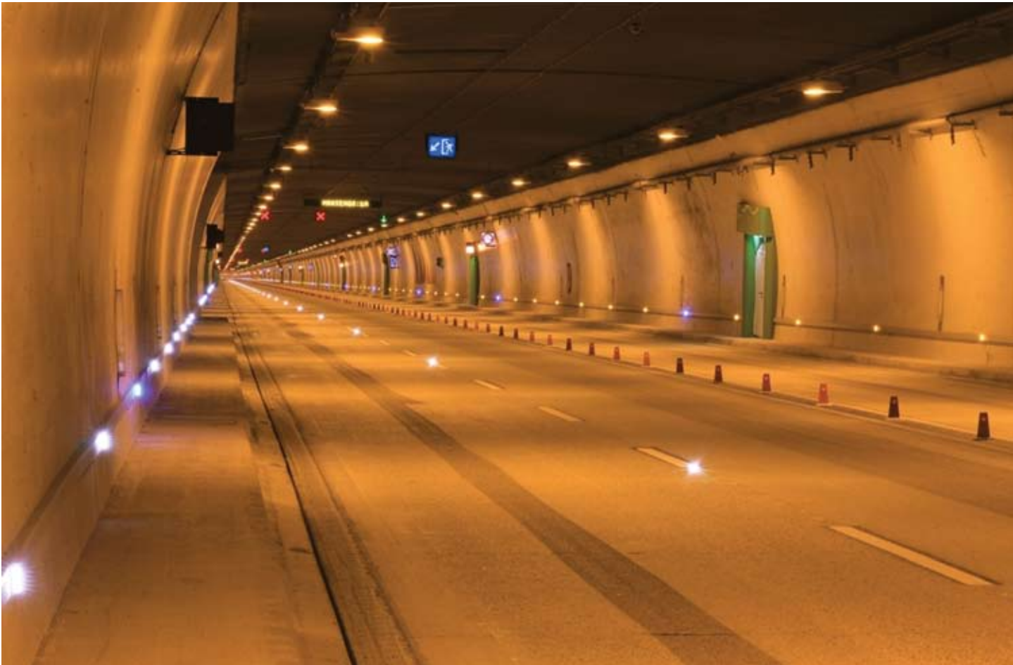
Figure 16: Juan Carlos I Tunnel (Spain)
