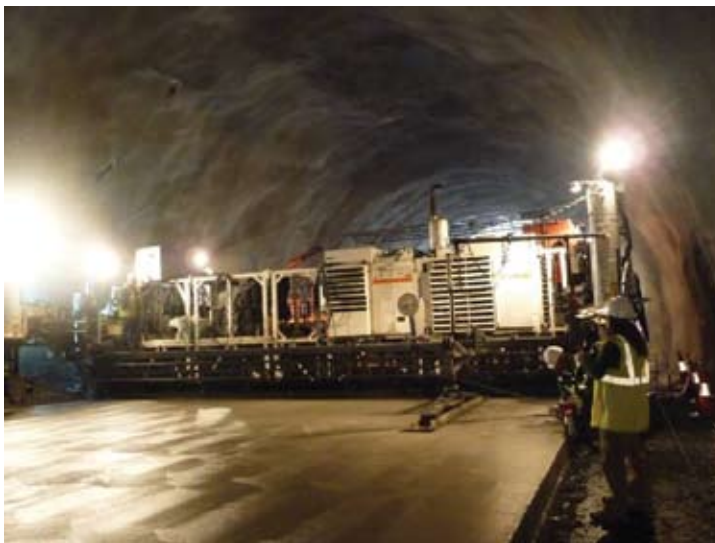
Figure 19: Construction by full width
