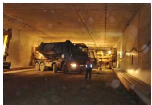
Figure 20: Side dump truck
