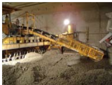
Figure 22: Two layer pavement: supply of concrete of the upper layer
