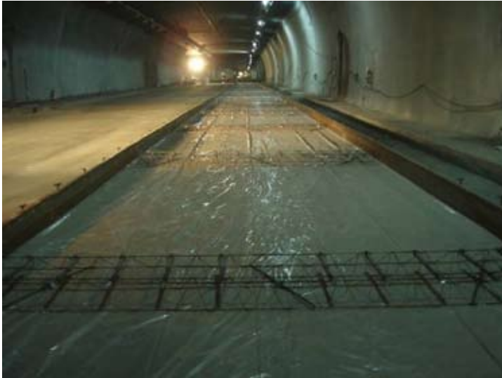
Figure 18: Construction by half widths
